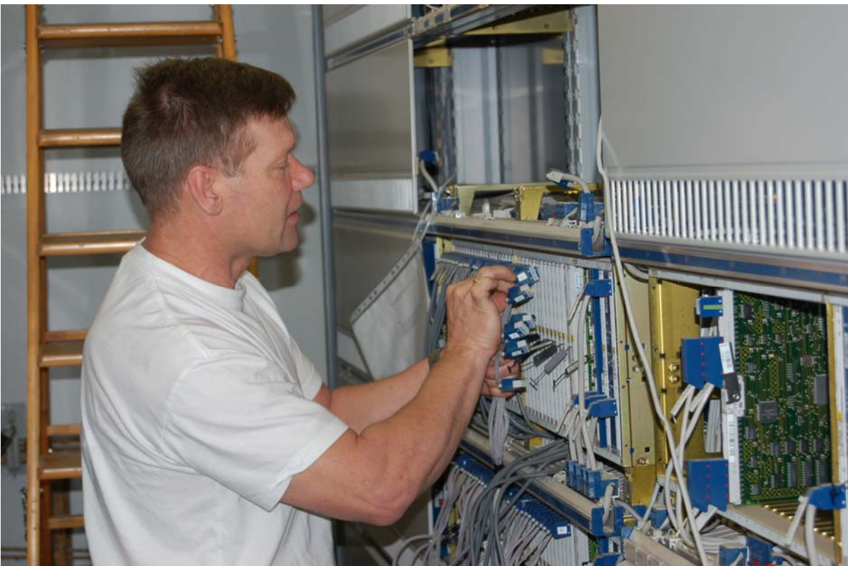
Mount eventually temporary cabling to MDF to maintain service during switchover
