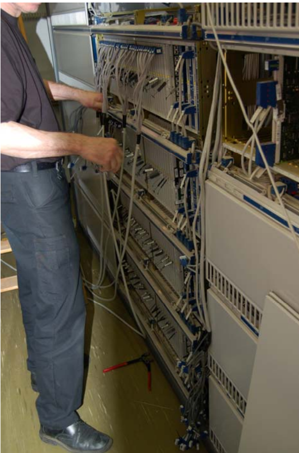
Temporary cabling mounted in MDF
