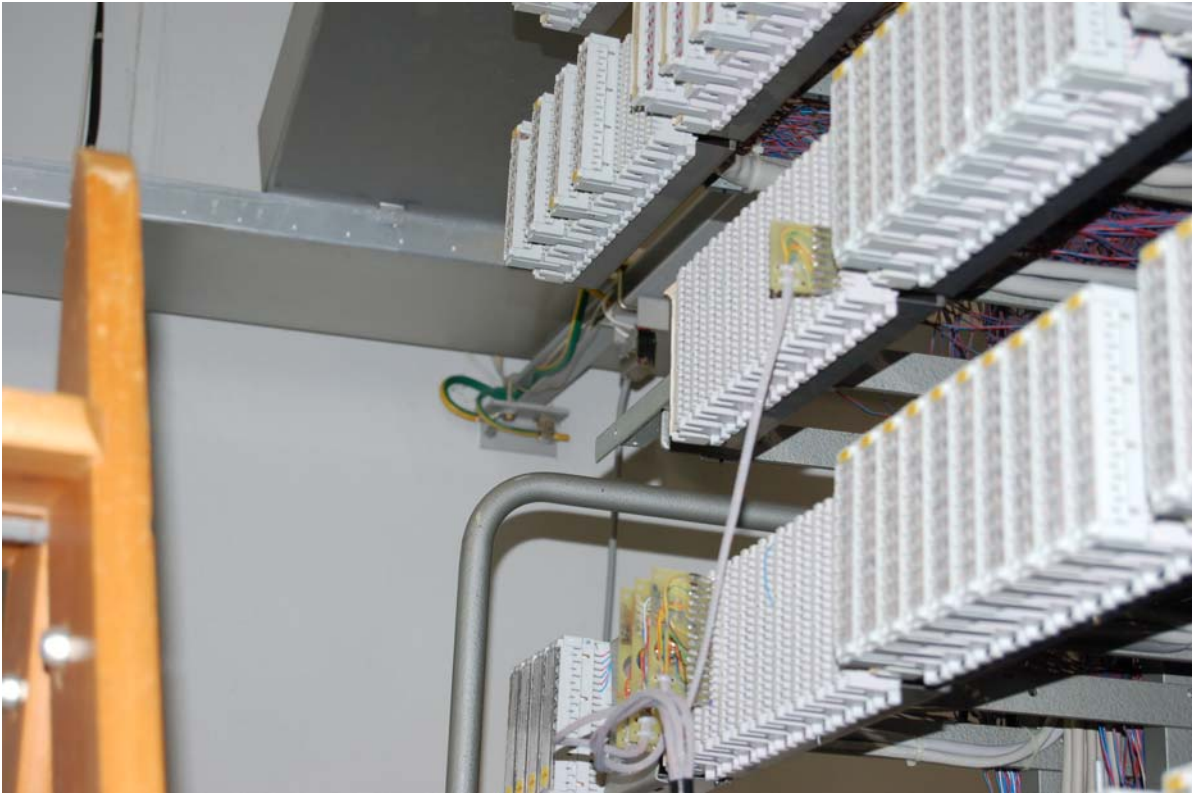
Temporary cabling mounted in MDF
